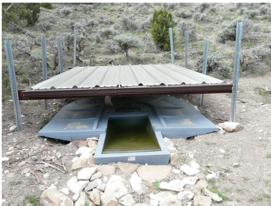
Figure 4. RotoGuzz brand guzzler with a metal apron constructed on top of the tank to enhance rain-gathering capability and increase protection
