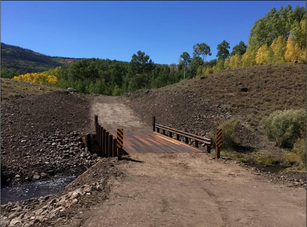
Figure 8. Bridge installed in 2019 to replace the ford crossing of Right Fork UM Creek at Black Flat.
