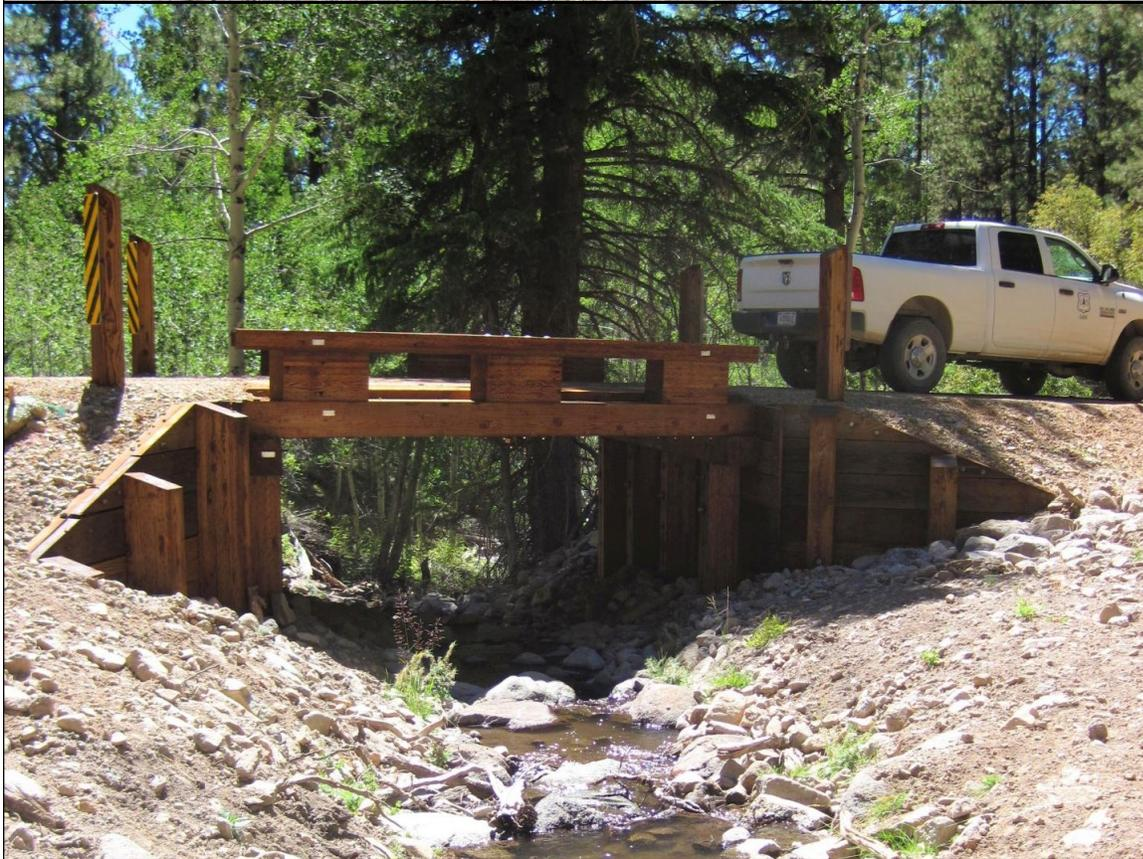
Figure 6. Fish-passable culvert (top) and timber crib bridge (bottom) that replaced previously impassable culverts in Hall Creek at Forest Highway 17 and the upper administrative road, respectively.
