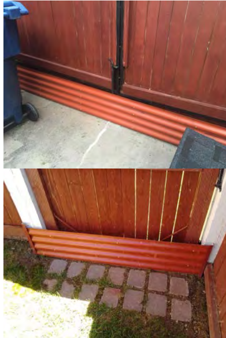
Figure 5. Installing a gate barrier is an important part of securing your backyard. When the gate is open, the barrier should act as a visual and physical barrier for the tortoise, but should be low enough (18") for people to step across. Gate barriers, if installed correctly, can be slid up and removed when moving large items into the yard (e.g., lawn mowers, garbage cans). (Photo by Desert Tortoise Group.)
